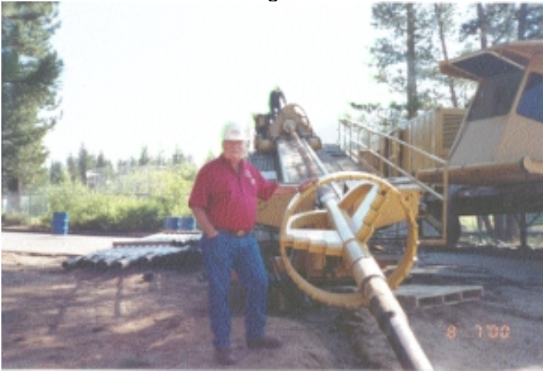
Figure 4 Fly cutter prior to the forward reaming
