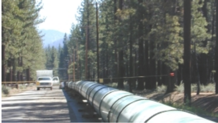
Figure 1 Welded and Coated Pipe String on Barbara Avenue
