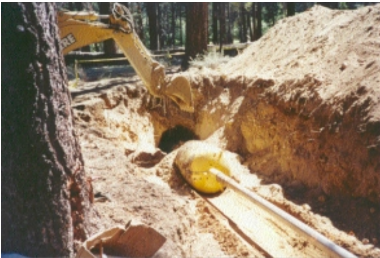
Figure 4 Fly cutter prior to the forward reaming
