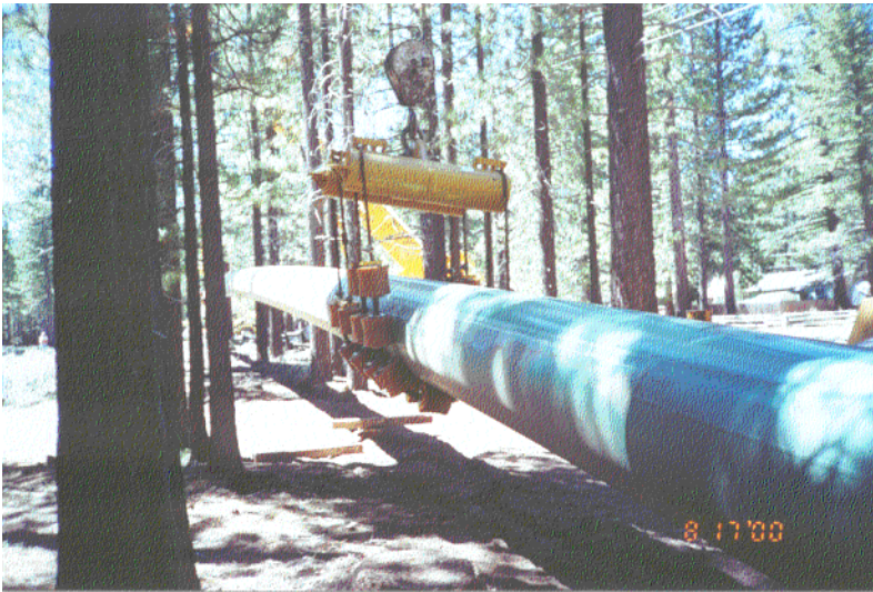
Figure 6 Pipe pull-back
