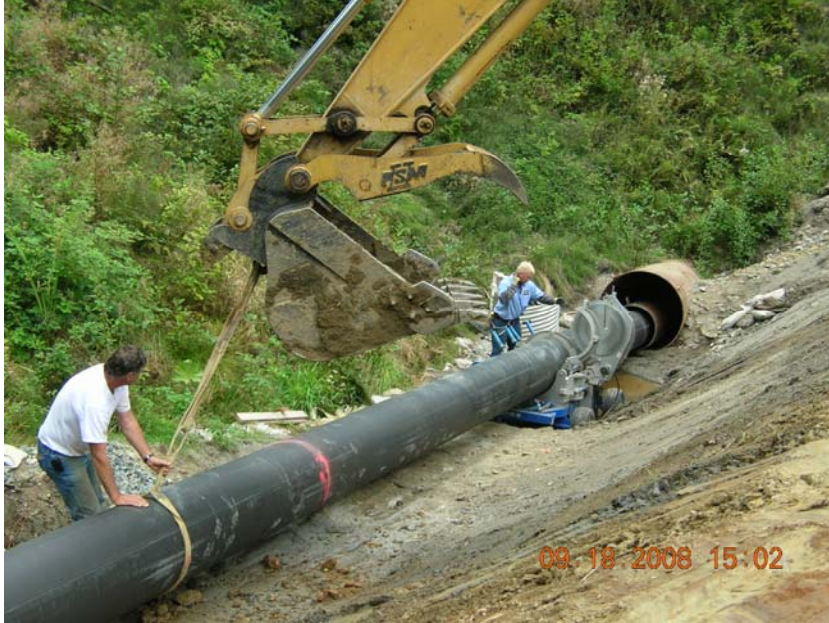
Figure 6: Installation of the 24-inch HDPE product pipe
