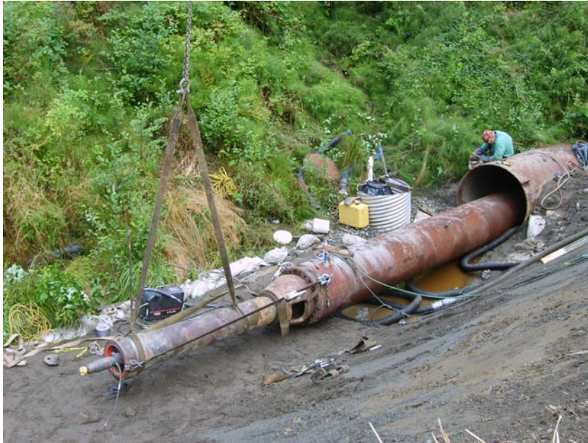
Figure 4: The Grundoram hammer ready to ram
