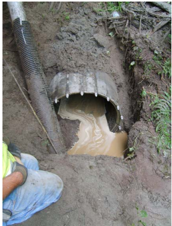
Figure 5: Daylight of the 30-inch casing. The bullet teeth can be seen around the edge of the cutting shoe.
