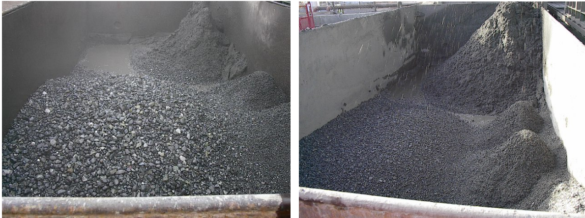
Figure 1 Spoil Bin with Significant Gravel (left) Spoil Transitioning to Fine Sand and Silt without Gravel (right)
