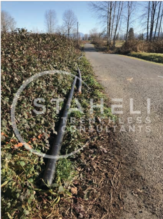
4" HDPE Pipe laid out prior to Pullback
