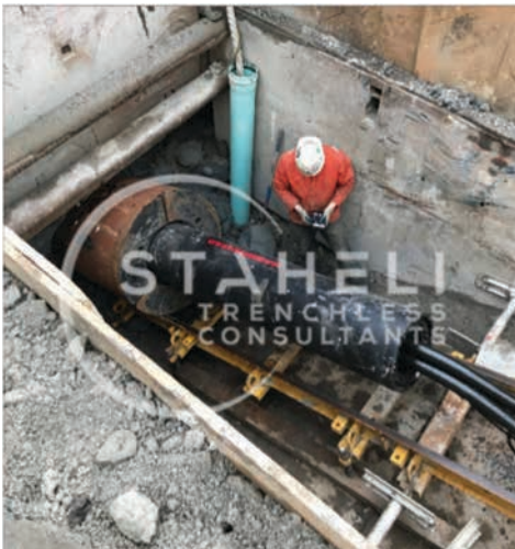
Pipe Ramming Installation of Conductor Casing
