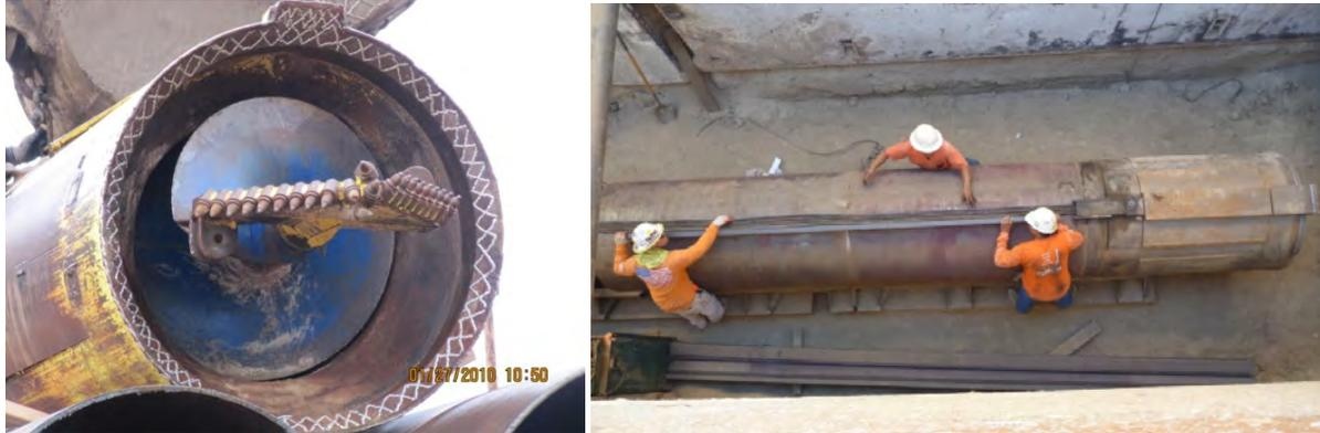
Figure 2. Steerable head with a hydraulic wedge at the 12 o'clock position (left). Steel "C" channel to protect the hydraulic lines and water level running along the top of the steel casing (right).
