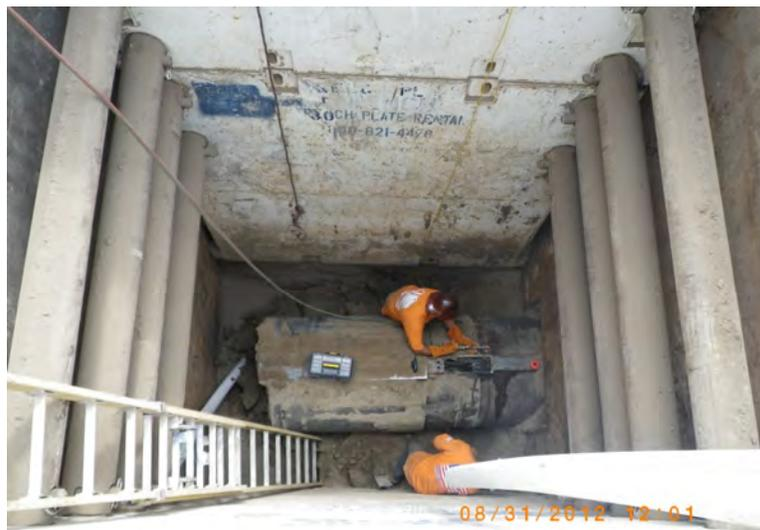
Figure 8. Steerable head being removed from the 42-inch casing within the reception shaft.
