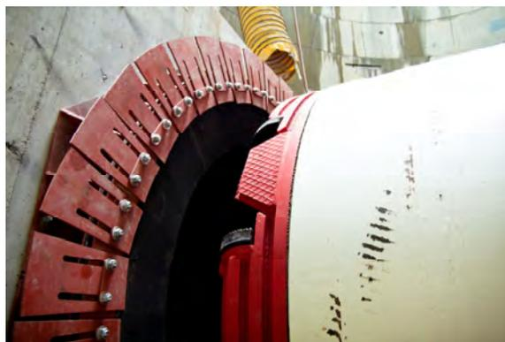
**Figure 4. Entry Seal Mounted to Shaft Wall for Launch**
