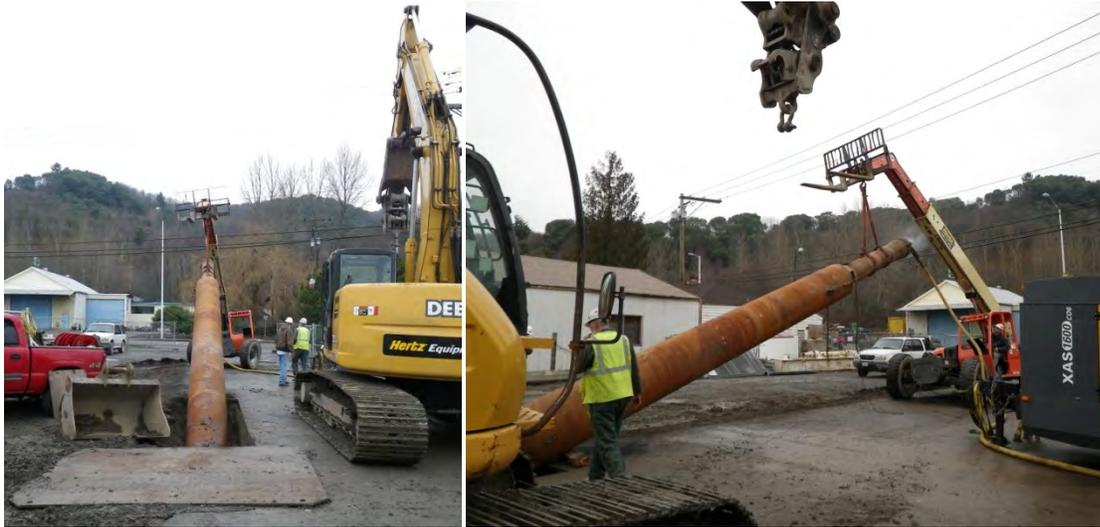
Figure 6. Installation of the 86LF entry conductor casing at 20 degrees.
