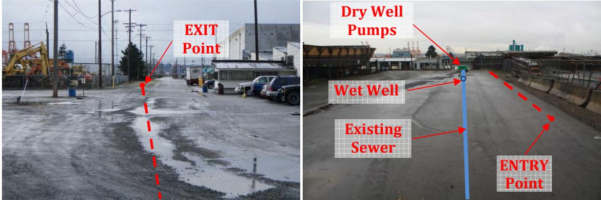
Figure 3. Exit Site View (left) and Entry Site View (right) with HDD alignment as dashed line.
