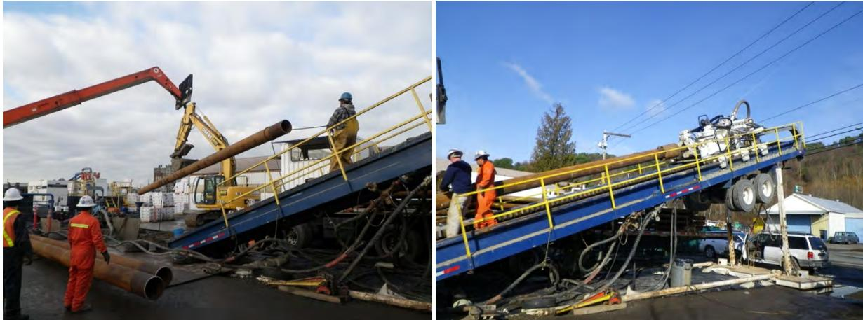
Figure 8. Installation of 120 feet of 12-inch wash over casing.
