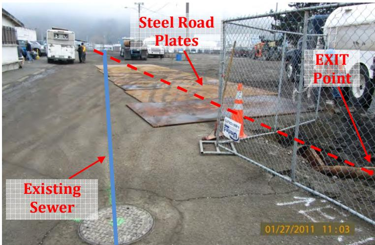
Figure 10. Exit Site with Existing Sewer and Steel Plates Over the Bore.
