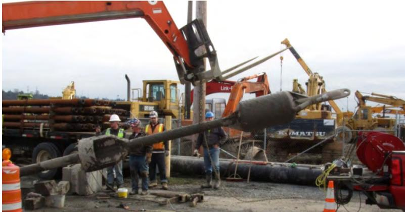
Figure 11. Fly cutter and barrel assembly used for back reaming.
