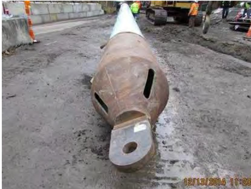
Figure 9. Slotted Pull Head to Allow Drilling Mud to Enter Pipe
