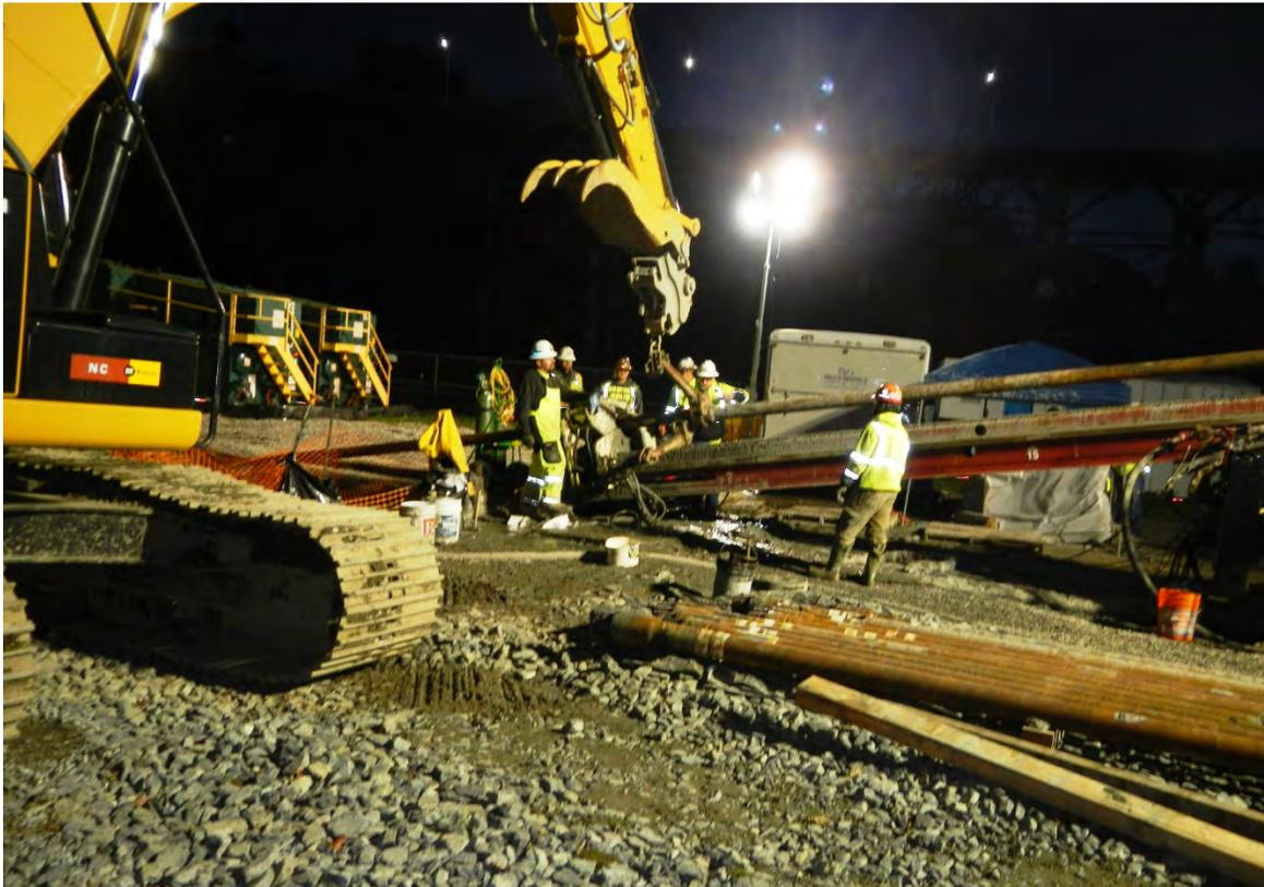
Figure 5. Drill Rig Set-Up in Smith Cove Park (lower end of the bore)
