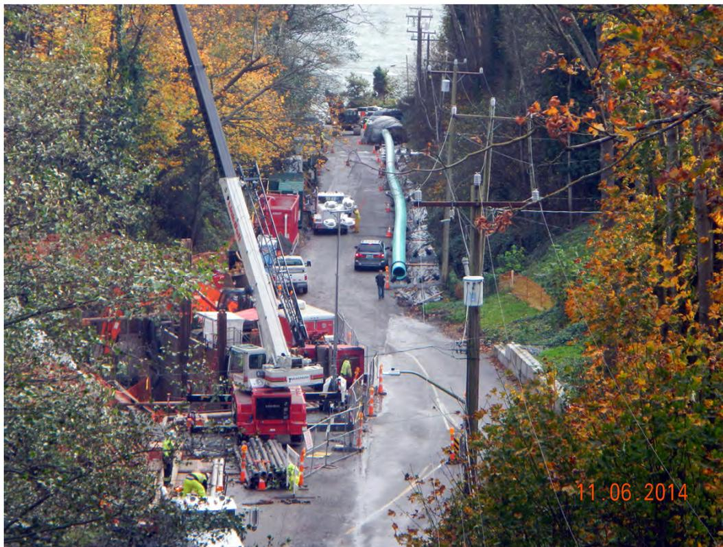
Figure 8. Assembling the FPVC on 32<sup>nd</sup> Ave West for Pullback
