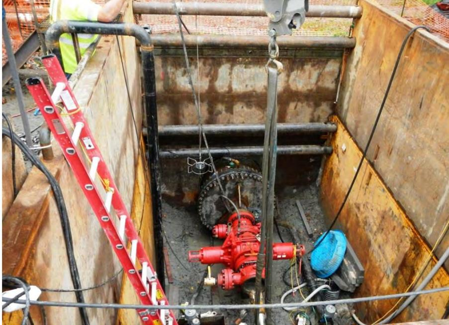
Figure 6. Blow-Off Preventer located in Shaft in Smith Cove Park
