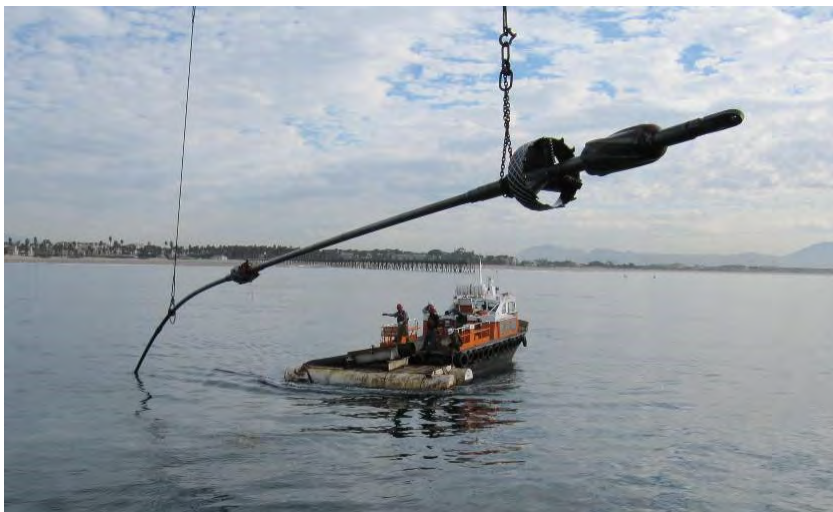
Figure 9. 48-inch reaming assembly exiting to the derrick barge
