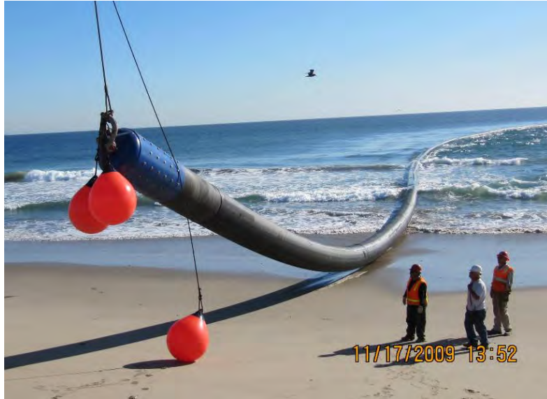
Figure 10. HDPE pipe heading out to sea from Pt. Mugu
