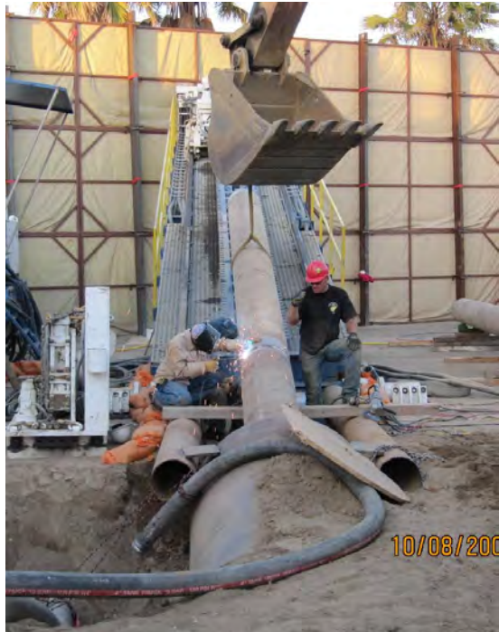
Figure 3. 18-inch centralizer casing installed in larger 54-inch casing
