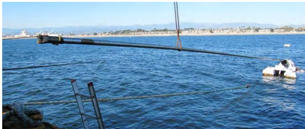
Figure 7. Drill string suspended between derrick barge and pontoon
