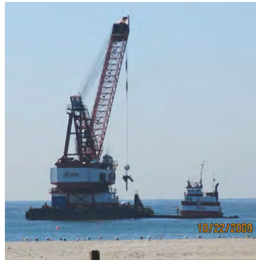
Figure 6. Derrick barge and supporting tugboat from shore
