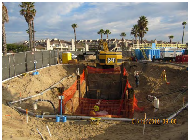
Figure 11. Excavation to expose pull head
