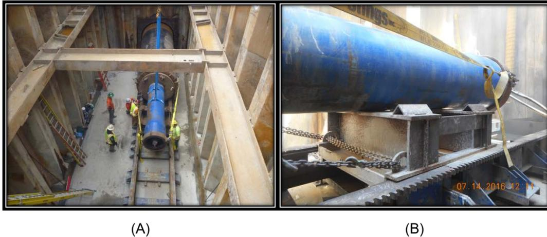
**Figure 6 (A) Grundoram Taurus pneumatic hammer. (B) Hammer Sled to hold hammer to design grade.**
