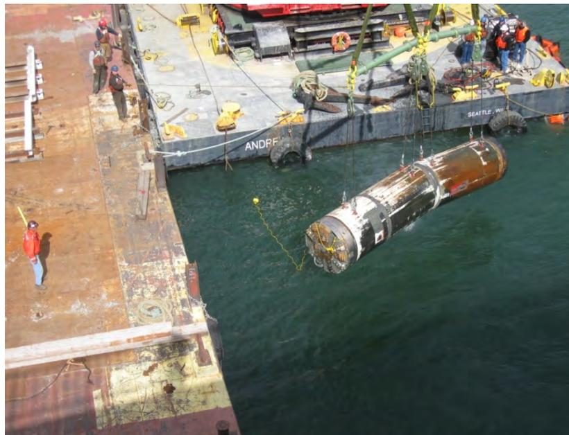
Figure 7. Wet Retrieval of MTBM
