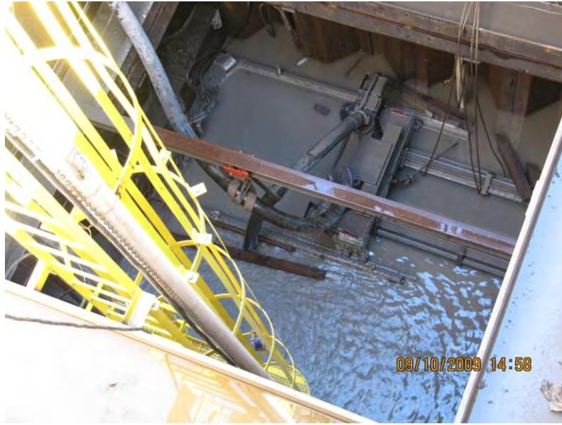
Figure 6. Flooded Shaft
