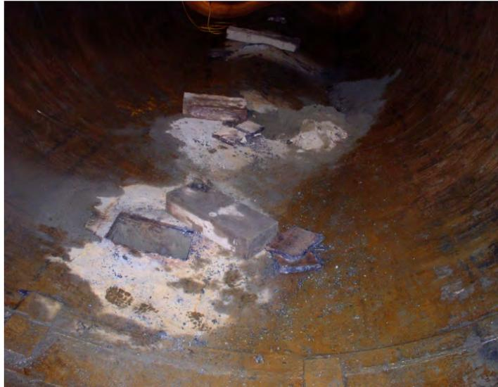
Figure 3. Exploratory Holes Cut into Casing Invert at Initial Point of Failure
