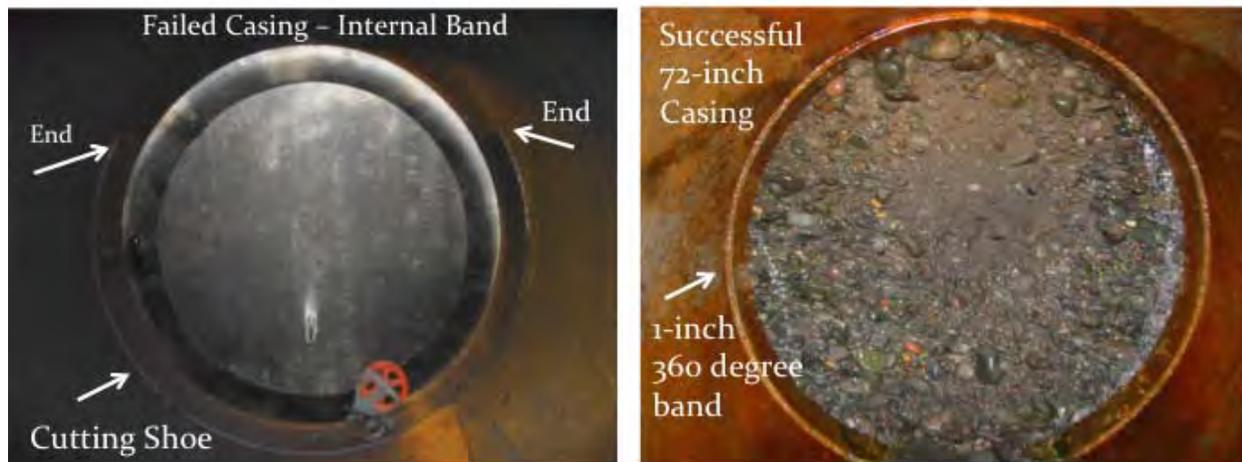
Figure 6. Partial Internal Banding (270 degrees) on the 120" casing (LEFT); Full Internal Banding used on successful 72" Pipe Ram in Dense Glacial Soils (RIGHT)
