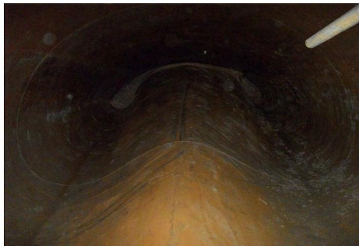
Figure 2. Casing Failure with Invert Deforming to the Crown of 144-inch Casing
