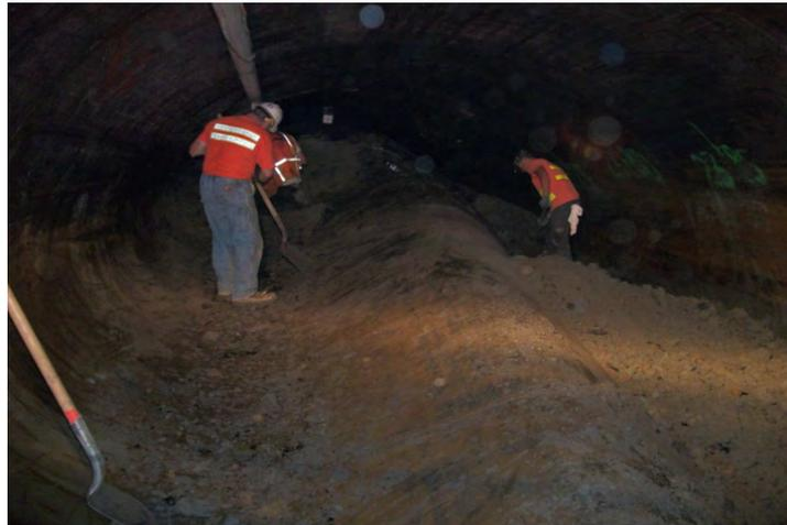
Figure 1. Invert Deformation of 144-inch Casing
