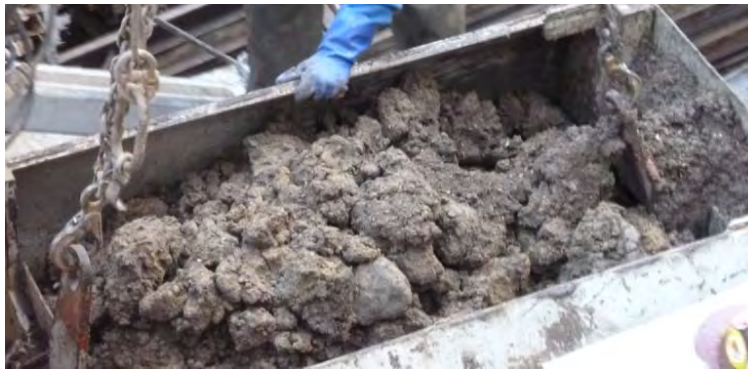
Figure 7. Fill Material Excavated During Open Shield Pipe Jacking
