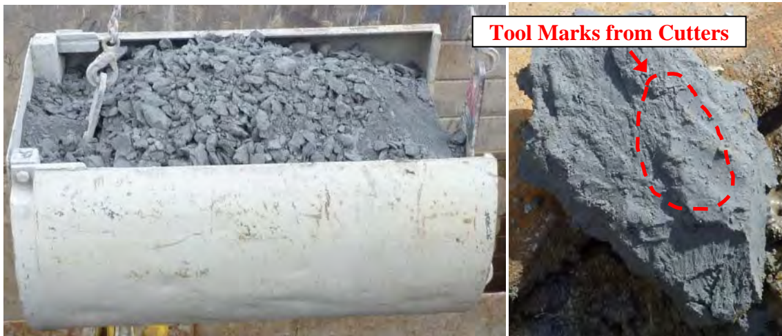
Figure 6. Very Stiff Lacustrine Spoils Excavated During Open Shield Pipe Jacking
