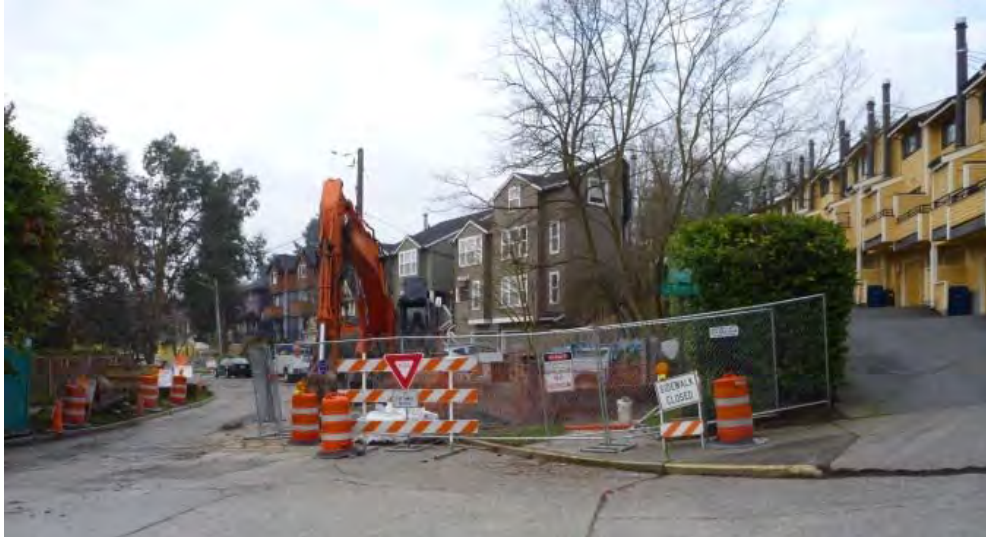
Figure 8. Reception Shaft Positioned in Neighborhood Street
