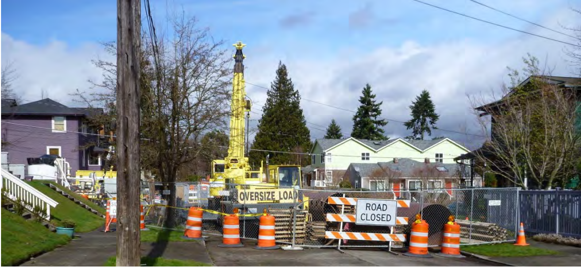
Figure 9. Constrained Jacking Shaft Site Overlooked by Adjacent Homes
