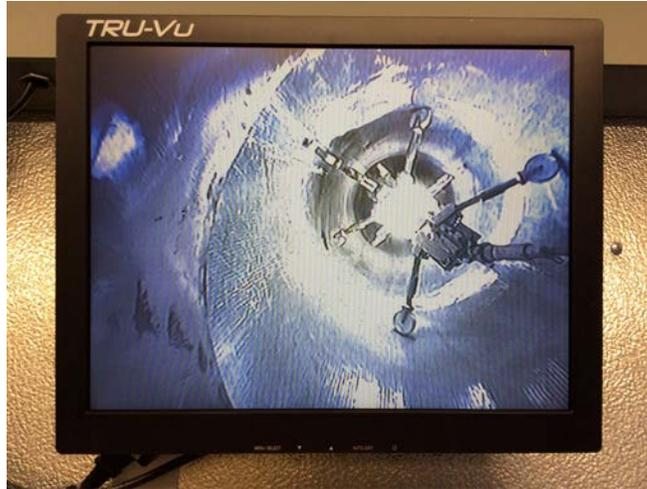
**Figure 3:** UV light Train Curing the 42” pipe on NE 112th & Holman
