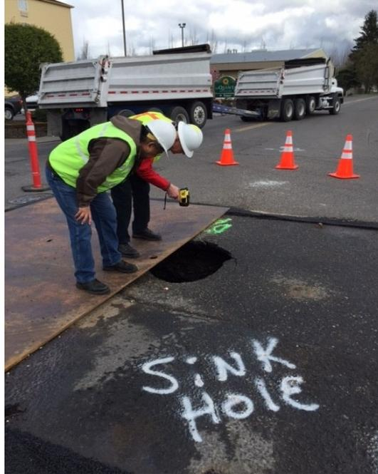
**Figure 1: Sink hole over failed 42" sewer requiring a quick repair**
