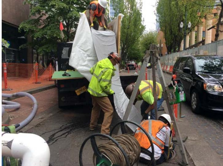
**Figure 5:** Inserting 10” UV CIPP Liner on SW Yamhill St. Located Underneath Train Tracks
