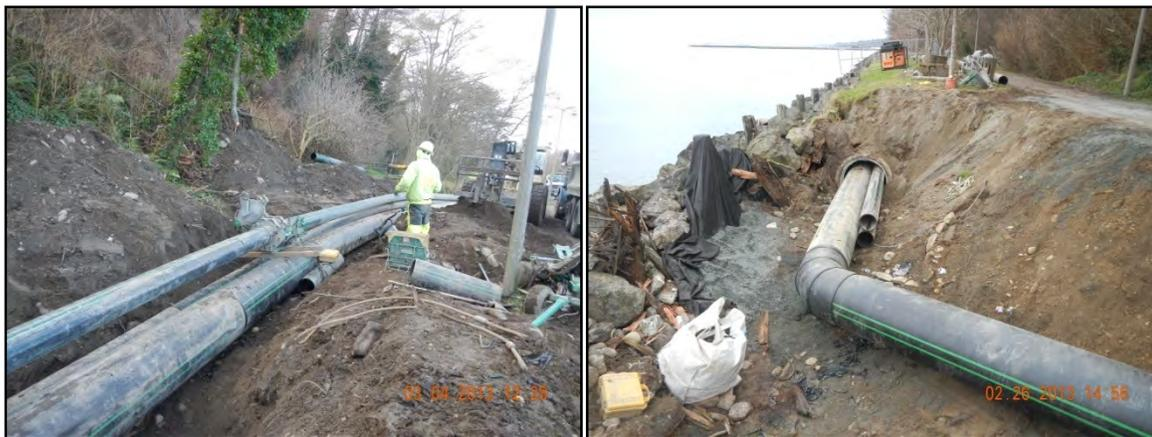
Figure 9. (Left) In-pit fusion of the 14-inch pipe. (Right) Fusion of the 30-inch pipe at an angle/elevation change.
