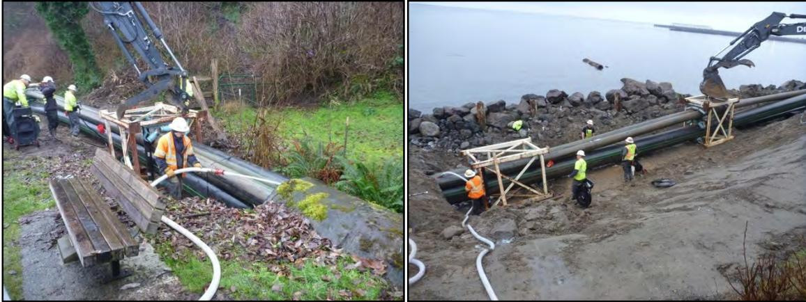
Figure 6. (Left) Pullback from pit C to B with liquid polymer lubricant. (Right) Pullback from pit F to D.
