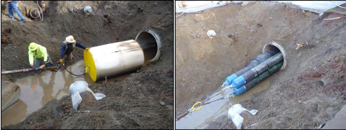
Figure 4. (Left) Proof and cleaning pig pulled prior to slipline. (Right) Test bundle pulled prior to slipline.
