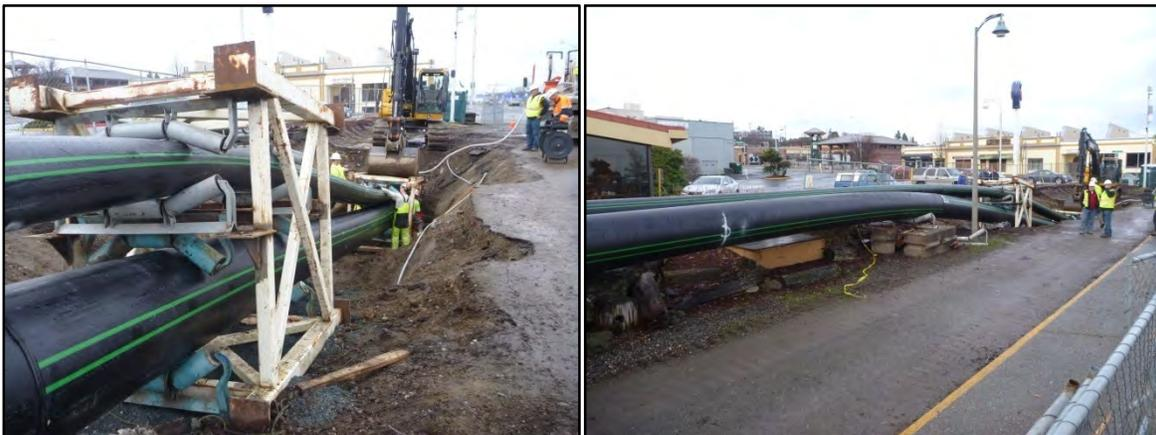
Figure 5. Insertion of 30-inch and two 14-inch pipes using bundling/taming frame.
