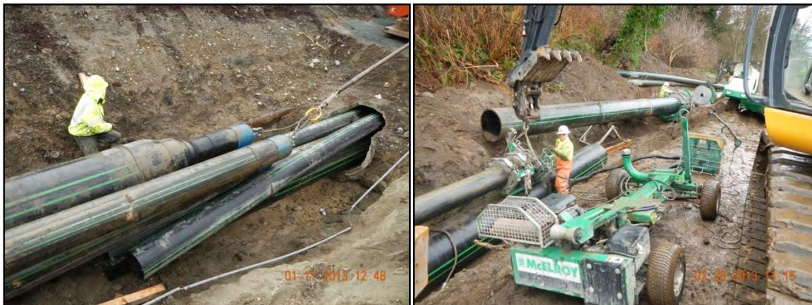
Figure 8. (Left) Slipline pit with two pipe bundles. (Right) In-pit HDPE fusion machines used to make connections.
