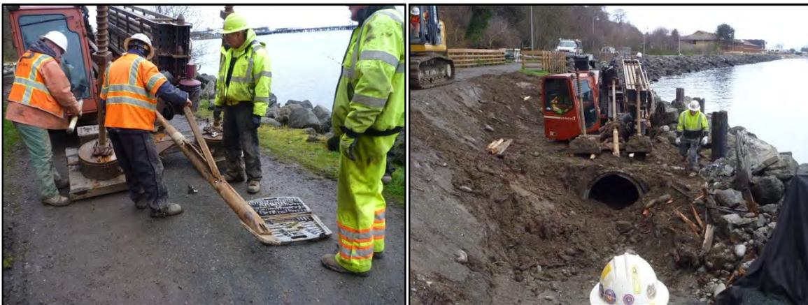
Figure 3. (Left) HDD battery powered locating sonde. (Right) HDD rig setup over existing host pipe.
