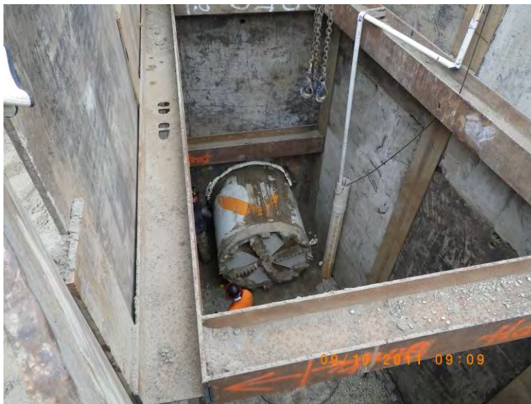
Figure 7. TBM entering the Reception Shaft
