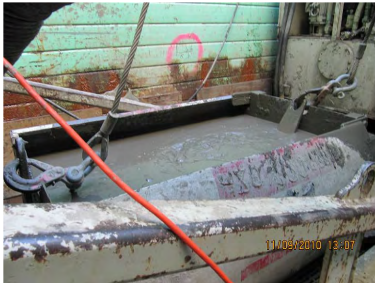
Figure 5. Saturated spoils in the muck bucket
