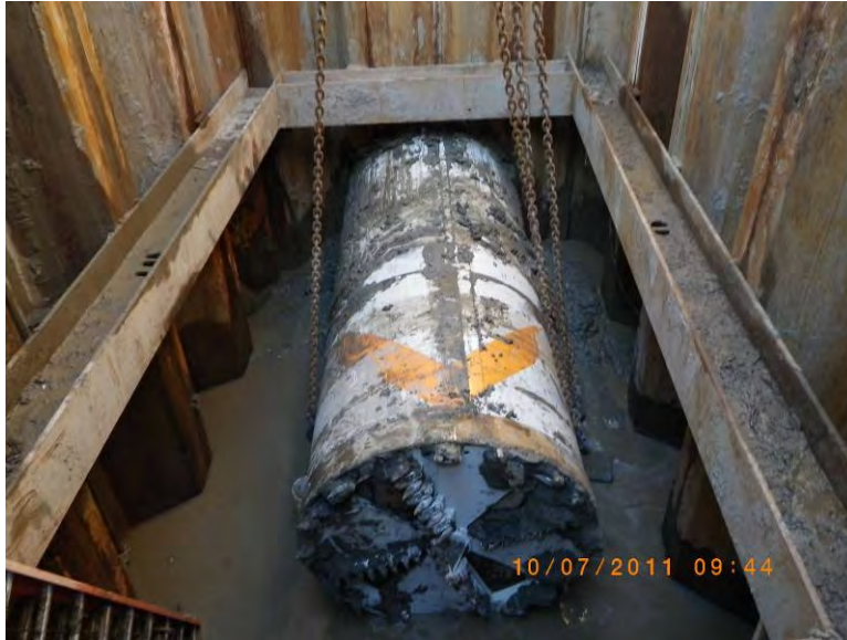
Figure 11. TBM being hoisted out of the Reception Shaft
