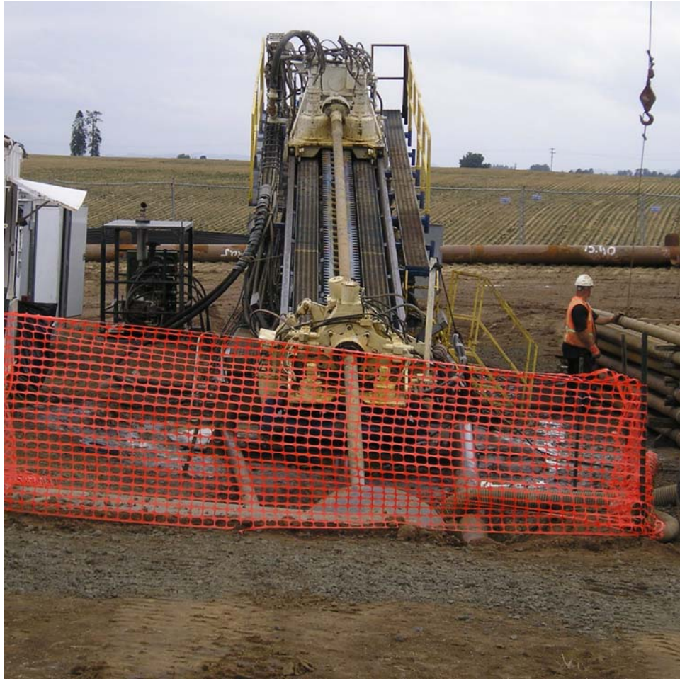
Figure 7 HDD Rig at the Beginning of the Pilot Bore.
